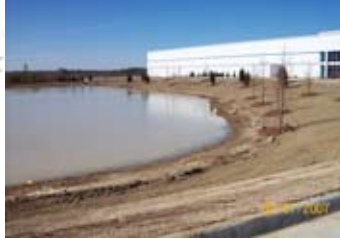
JDA Building Isle of Wight, VA
