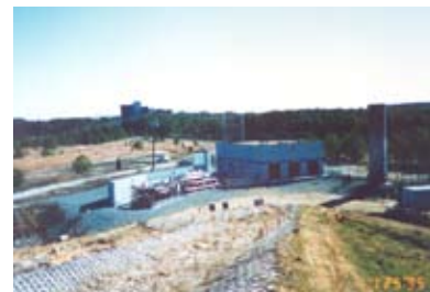
Landfill Gas to Energy
