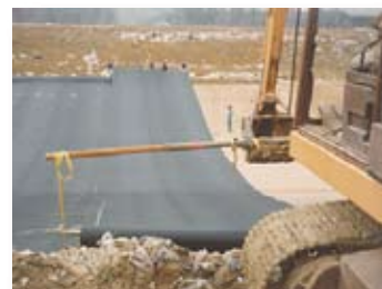
Membrane Liner Installation King William County, VA
