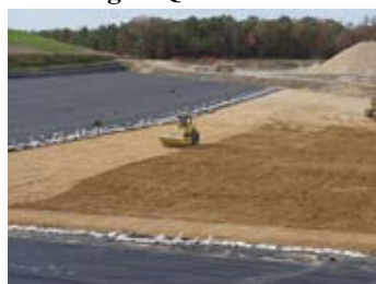
Liner Installation Ashcake Road Landfill
