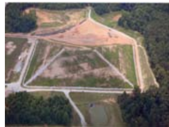
Landfill Closure Prince Edward County, VA
