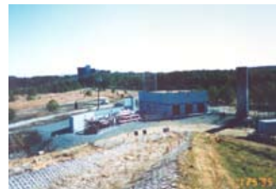
Landfill Gas to Energy
