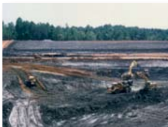
Lining Subgrade King & Queen Landfill
